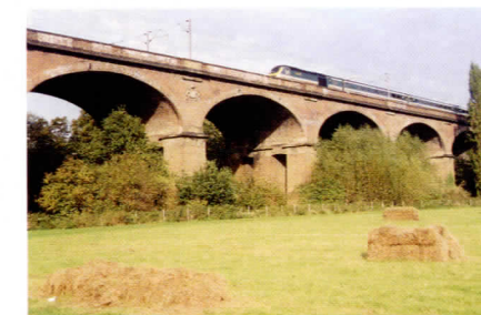
The 275-metre long Wharcliffe Viaduct still carries London-Bristol trains at an elevation of almost 20 metres across the Brent Valley in West London.
